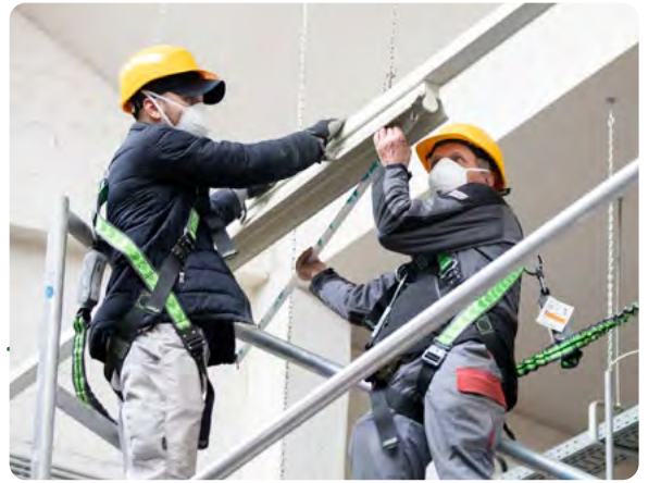
Removal of fluorescent tubes at VILLAGE IM DRITTEN, Vienna (2021, ARE Austrian Real Estate) © Anna Rauchenberger
