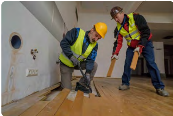
Removal of parquet flooring at MedUni Campus Mariannengasse, Vienna (2019-2020, Bundesimmobiliengesellschaft) © Harald A. Jahn
